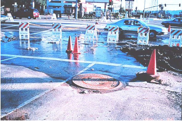
Fig. 2. Potable water leakage in the San Fernando valley after the Northridge earthquake, in January, 1994.
