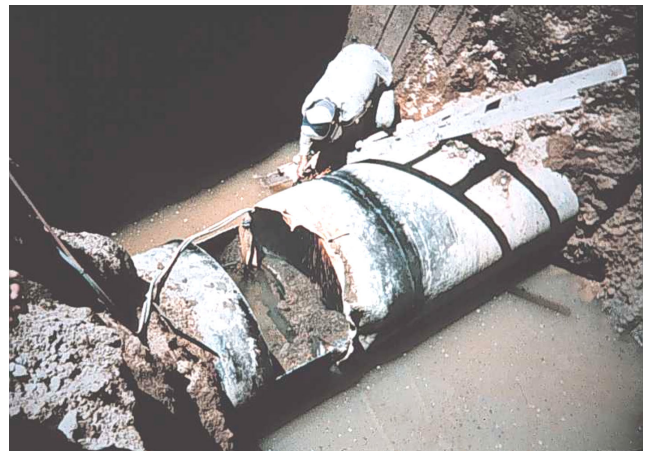
Fig. 6. Failure of a steel pipeline; Mexico City earthquake, 1985.
