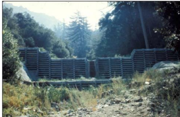
Figure 7. Debris basin constructed of precast concrete sections (Bradley et al. 2005)
