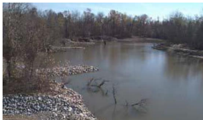
Figure 8. Weirs on outer bank of river (Bradley et al. 2005)
